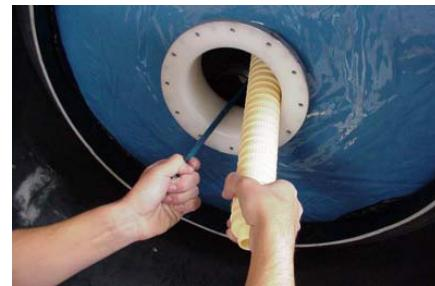
Step 3: Put assembly inside the tank to mount laterals.
