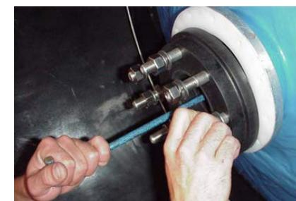
Step 5: Screw flange adaptor on assembly. Be sure O-ring is attached and sealed properly to adaptor.
